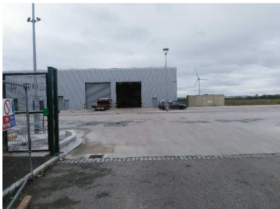
Plate 15- Industrial type shed & service yard
