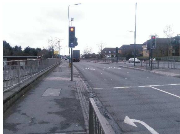
Plate 27 – Northend Road at Colyers Lane junction (facing south)
