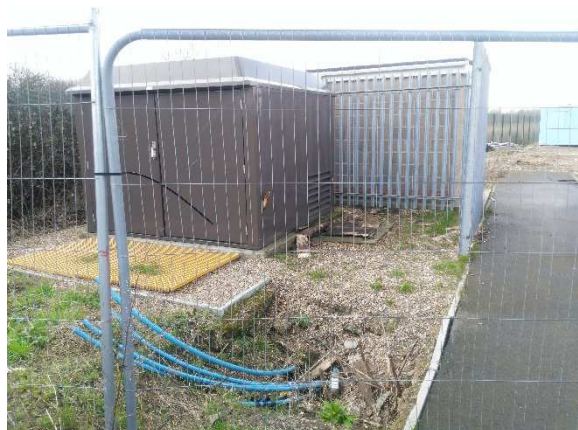
Plate 16 – New substation in southern corner
