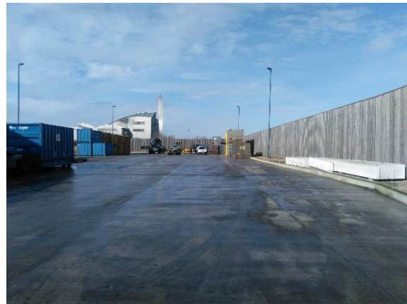
Plate 2 – Ash Container Storage Area
