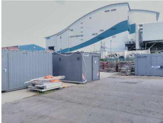
Plate 7 – RRRF Maintenance Depot
